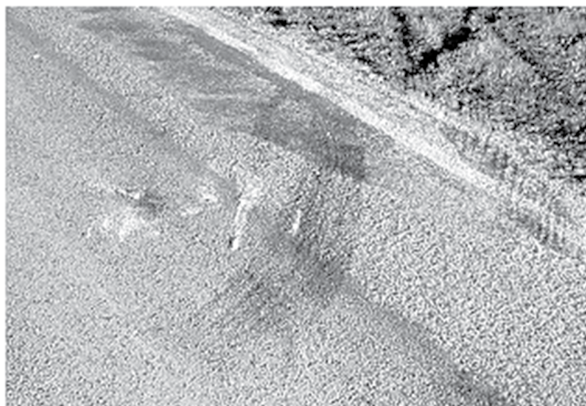
FIGURE 36 Example of scuff marks (broad, dark, sweeping marks on the roadway surface) and gouge marks (light-colored marks into the surface).
