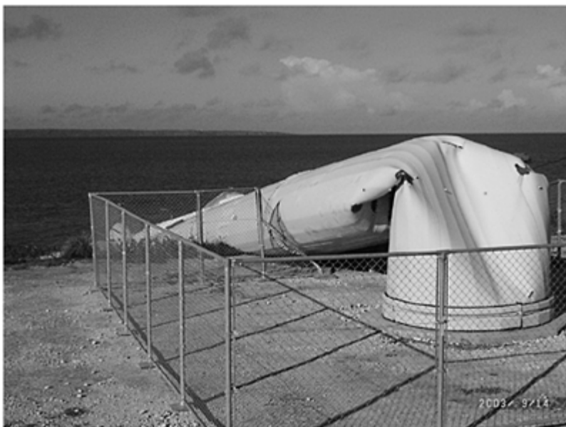
Figure 11.6 A failed wind turbine tower following a typhoon (picture by Dr M.Matsui, Tokyo Polytechnic University).
