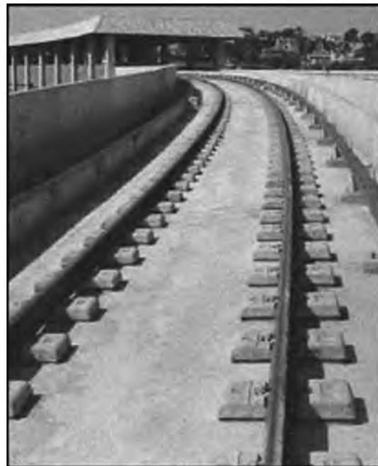
**Fig. 18.5** Low vibration track (See also Color Plate 15)
