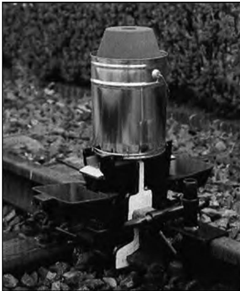
**Fig. 9.3** A Single Use Crucible (See also Color Plate 3)
