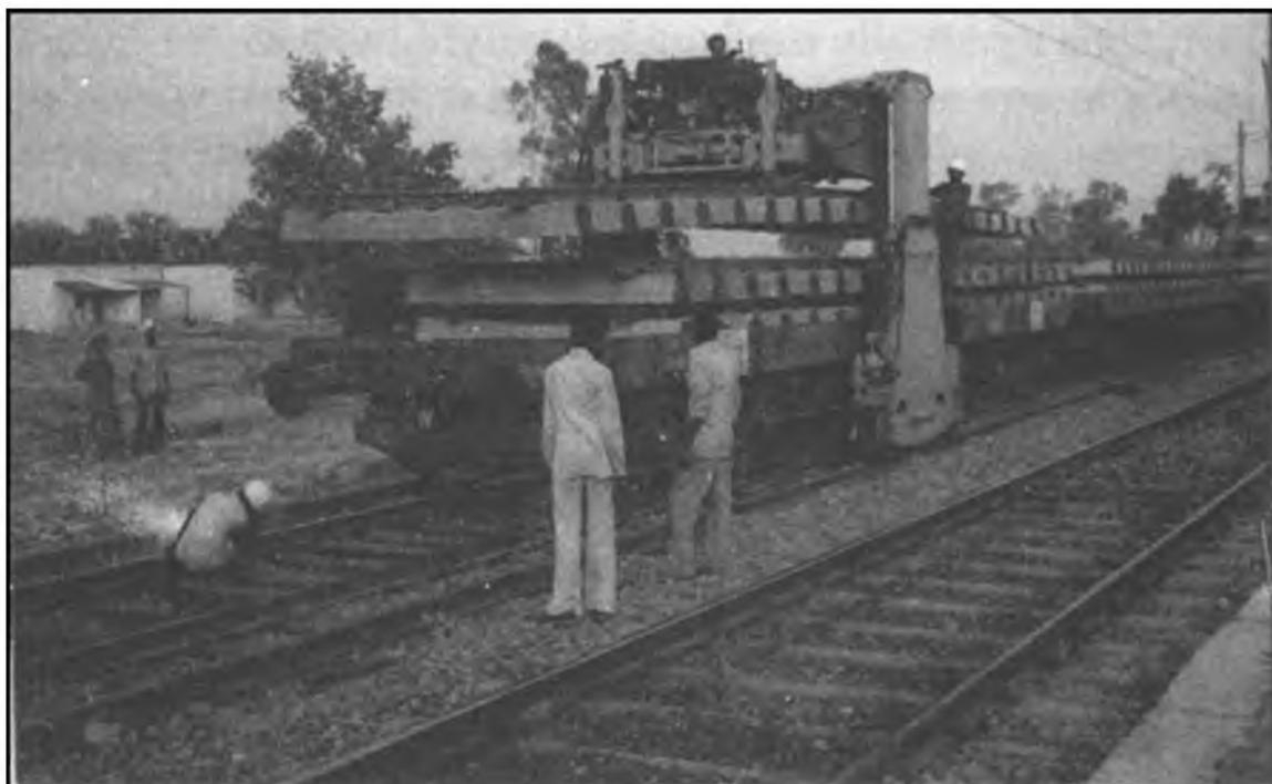
**Fig. 15.4 (b)** Portal crane licking up concrete sleeper panel
