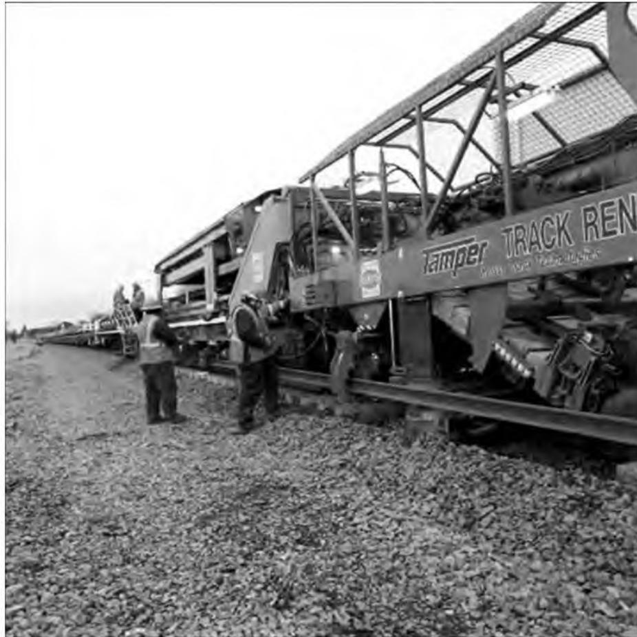
**Fig. 15.9** Picking of old sleepers and laying of new sleepers
