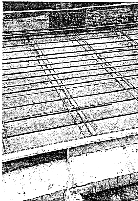
Figure 9.26: Steel reinforcement of the slab
