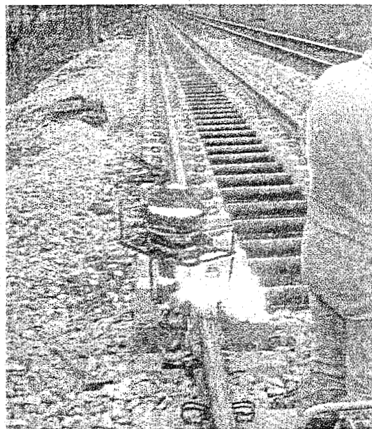
Figure 12.77: Thermit weld at beginning of renewal;
