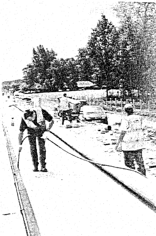
Figure 9.52: Pouring of the compound into the groove
