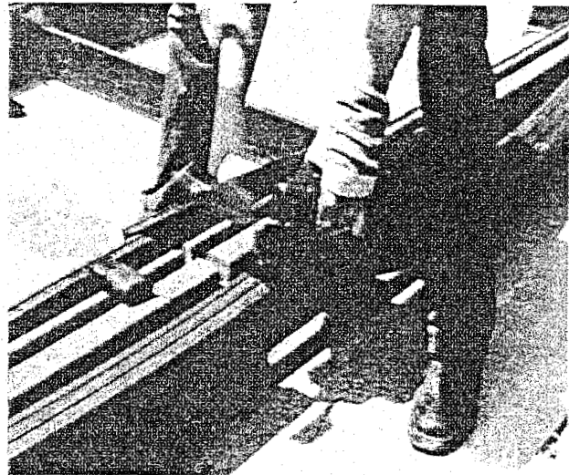
Figure 9.68: Fitting of the rubber chamber elements
