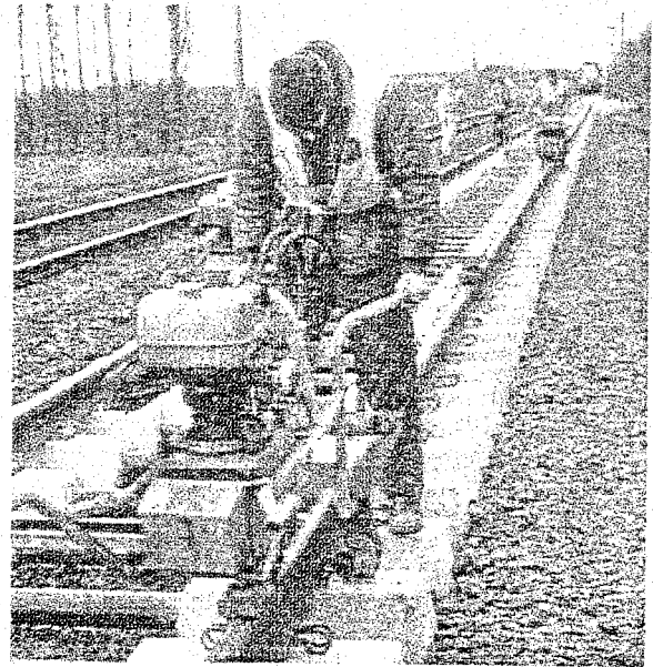
Figure 12.81: Fixing DE spring clips;
