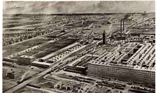
Hình 4.43: Western Electric's Hawthorne Work
